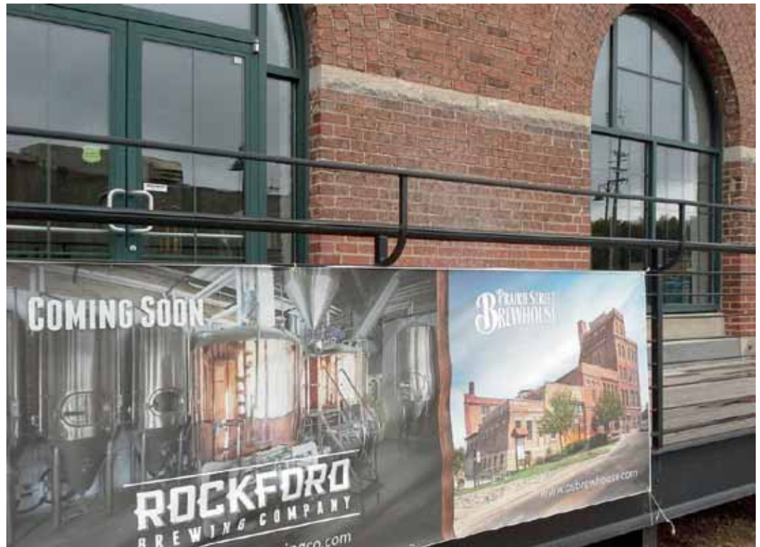
Rockford: Peacock Brewery rehabilitation
