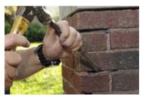
Hand chiseling is the method least likely to cause damage to the brick or stone. Removing mortar with saws, grinders,
