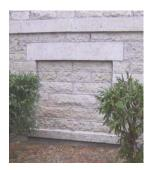
On masonry buildings, when original windows are closed-in, the infill material should match that of the wall and should be inset from the face of the wall at least two inches. Non-original windows can usually be closed flush to the wall surfaces with
