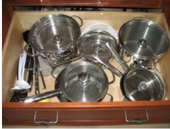
Figure 13 Example of a large drawer with full extension drawer slides
