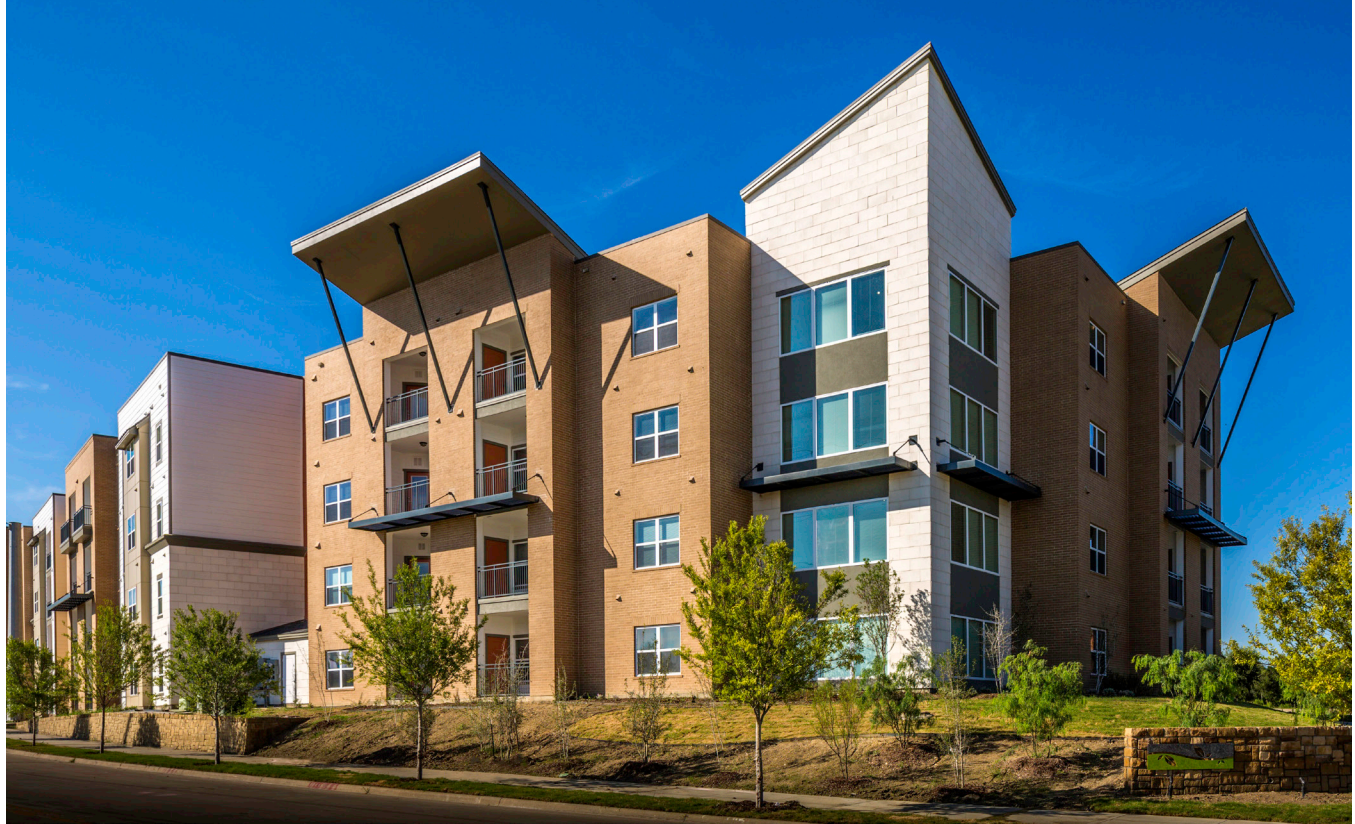
Photo: Courtesy of GroundFloor Development
