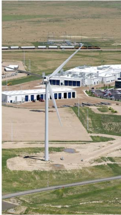
Tower factory (Pueblo, CO)
