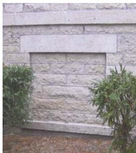
On masonry buildings, when original windows are closed-in, the infill material should match that of the wall and should be inset from the face of the wall at least two inches. Non-original windows can usually be closed flush to the wall surfaces with
