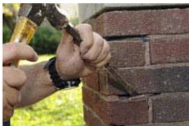
Hand chiseling is the method least likely to cause damage to the brick or stone.
